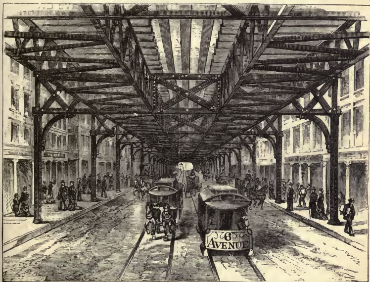
UNDER THE ELEVATED RAILWAY.
